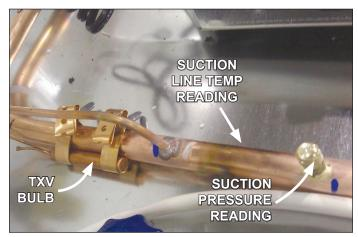
Fig. 16 Obtain pressure and temperature readings
