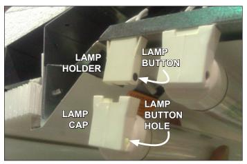
2. Attach the lamp caps and plastic shield to the new T-8 lamp.
