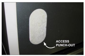
Fig. 10 Penetrate foam as needed to access piping
