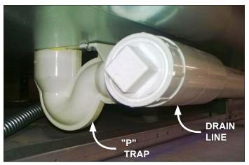
Fig. 12 "P" trap; drain line
