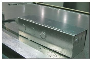
Fig. 14 Junction box on top of case
