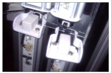
Fig. 21 Squeeze the latching clips and pull the luminaire free
