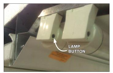
Fig. 18 Align new T-8 with plug button to secure
