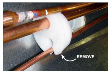
Fig. 11 Remove the shipping blocks
