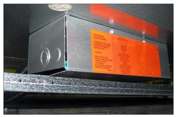
Fig. 13 Junction box beneath case
